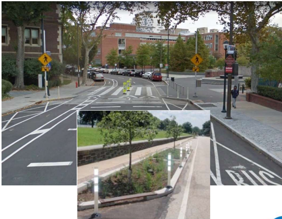
Stormwater bump-outs provide the pedestrian crossing benefits of curb extensions and help manage stormwater overflow.
